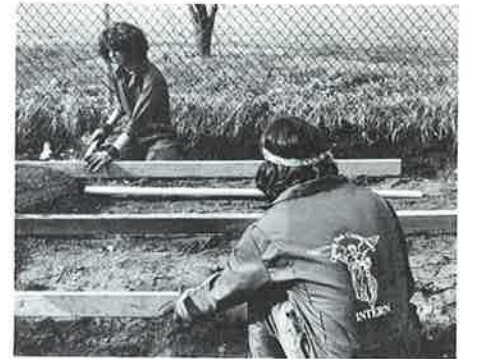
Central Park Conservancy interns rebuilding the Lilac Walk
